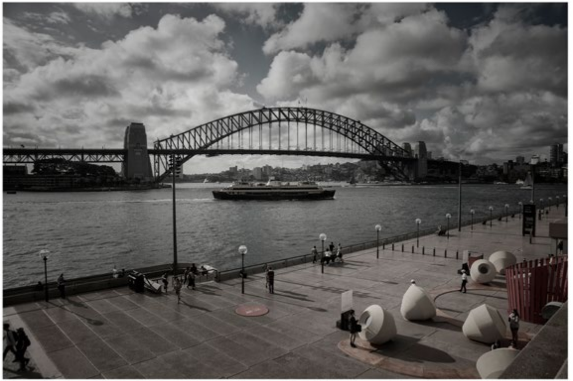
Sydney Harbour Bridge
