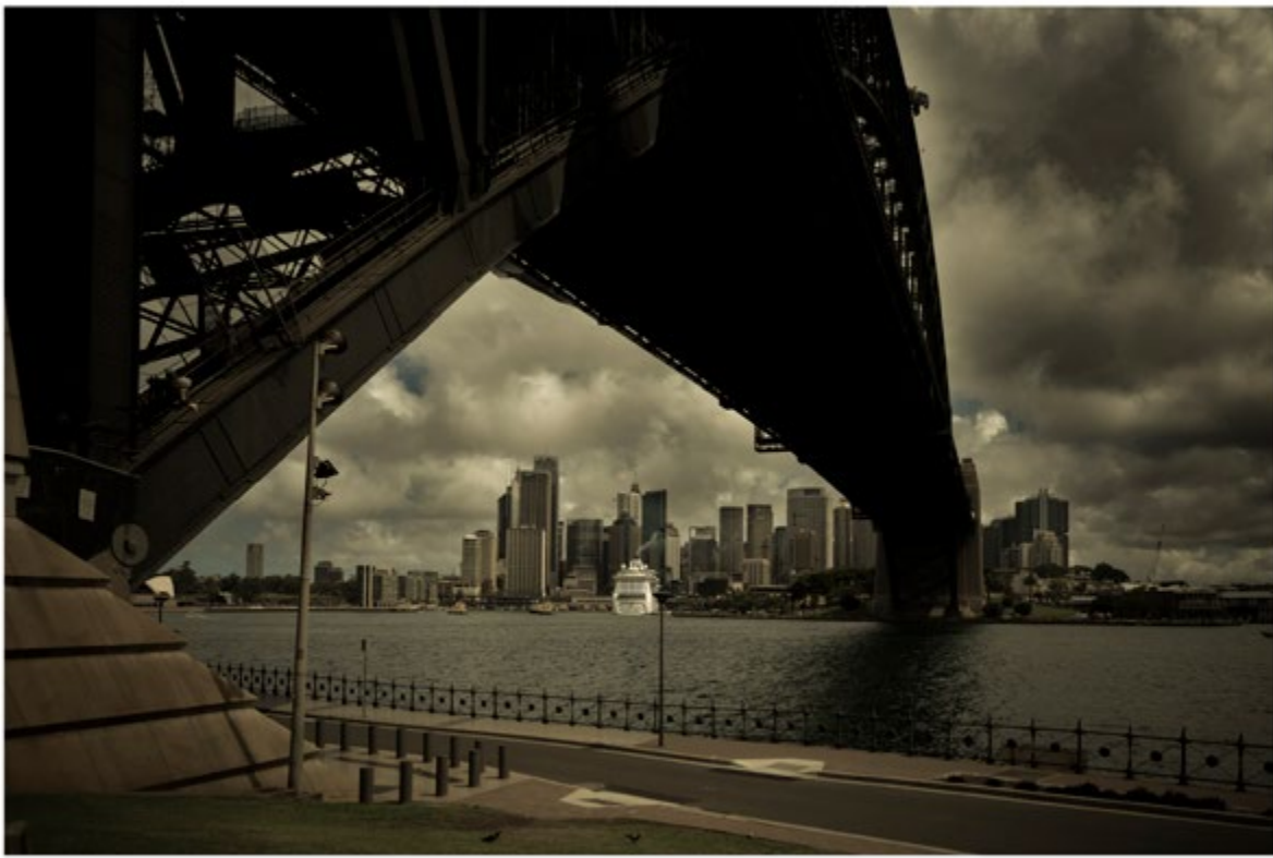
Sydney Harbour Bridge
